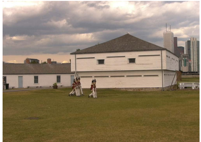
General View of the Blockhouse, Historic Fort York, Toronto, Ontario, August, 2006.
