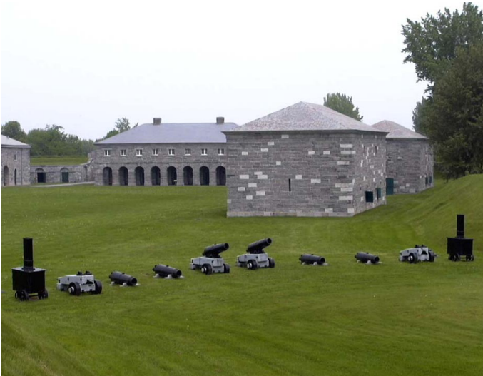
Stone Buildings & Ordnance, Fort Lennox National Historic Site, Île-aux-Noix, Québec, June, 2007.
