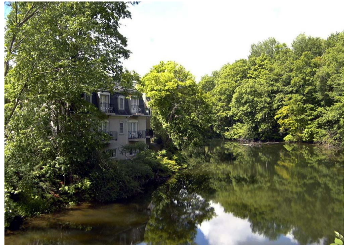
Rear of Gledhill House, a Benmiller Inn & Spa Annex Building near Goderich, Ontario, July, 2007.
