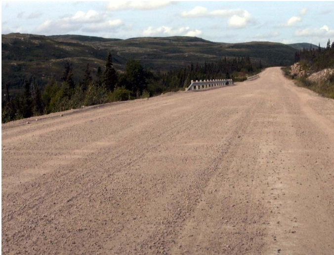
The Gravel Surface Section of Hwy. 510 between Red Bay and Lodge Bay, NL, September, 2008.
