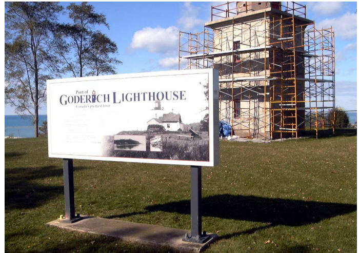
Scaffolding Surrounds the 1847 Lighthouse Ready for its Rehabilitation, Goderich, ON, October, 2009.
