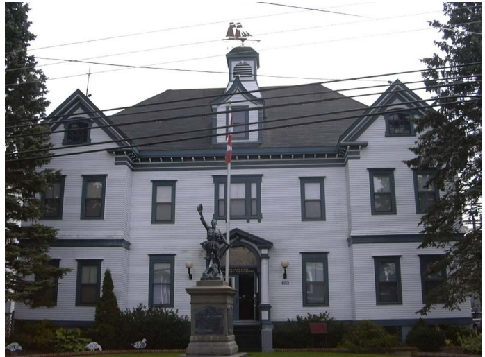
Exterior of Town Hall and War Memorial, Liverpool, Nova Scotia, September, 2009.
