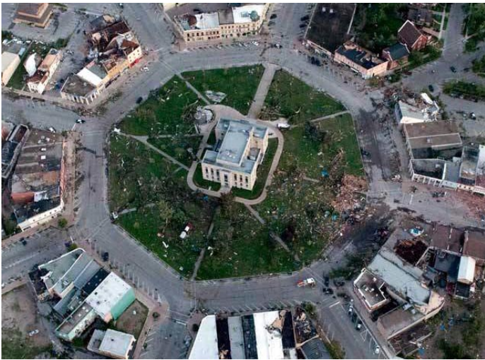
Destruction Caused to West Street, The Square and Court House, Goderich, Ontario, August 21, 2011.
