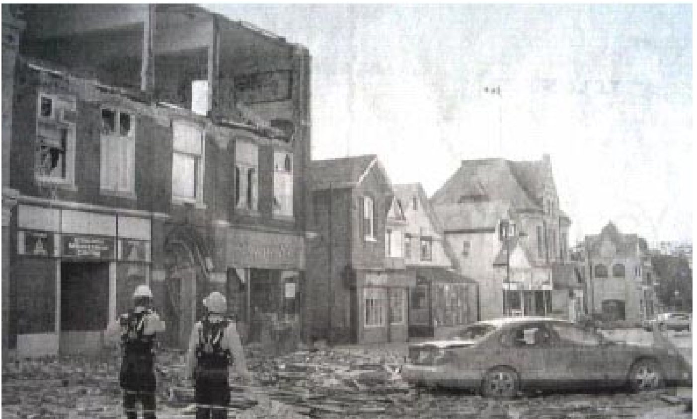
The Top of West Street Showing the Destroyed Façade of the Masonic Building, and Rubble Strwn across the Road. A Scene Reminiscent of a War Zone.
