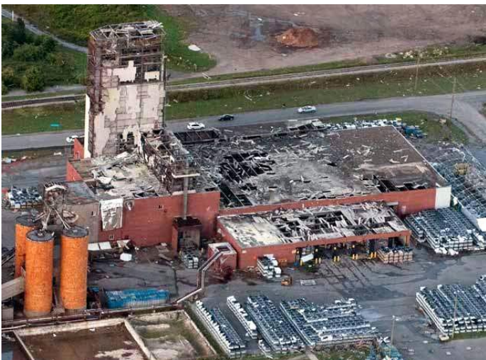
Destruction Caused to the Sifto Salt Evaporator Plant, Goderich, Ontario, August 21, 2011.
