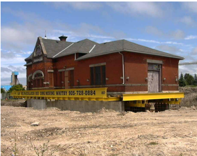
Moved CPR Station Resting on its New Foundations, Goderich, Ontario, August, 2013.
