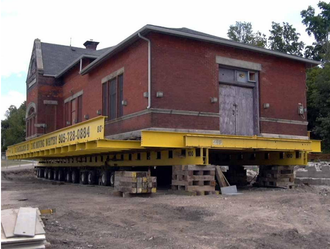
Moving of the CPR Station Using Wheeled Bogies, Goderich, Ontario, July, 2013.
