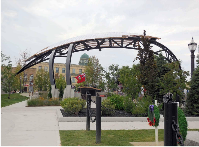
Newly Installed Performance Stage in Courthouse Park, Goderich, Ontario, August, 2014.
